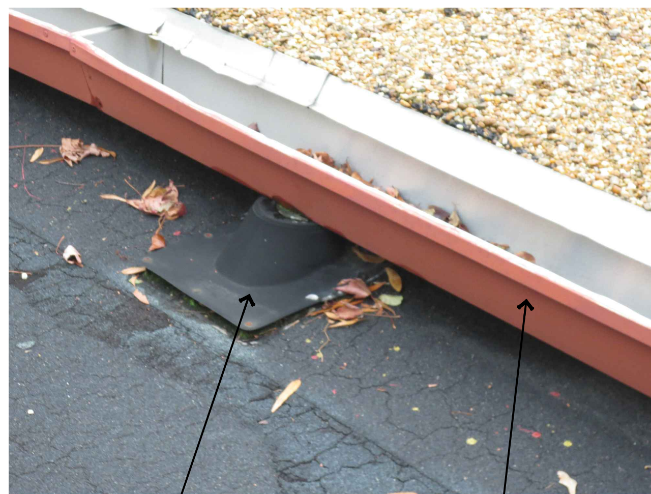
5 LOW ROOF TO MAIN ROOF TRANSITION
